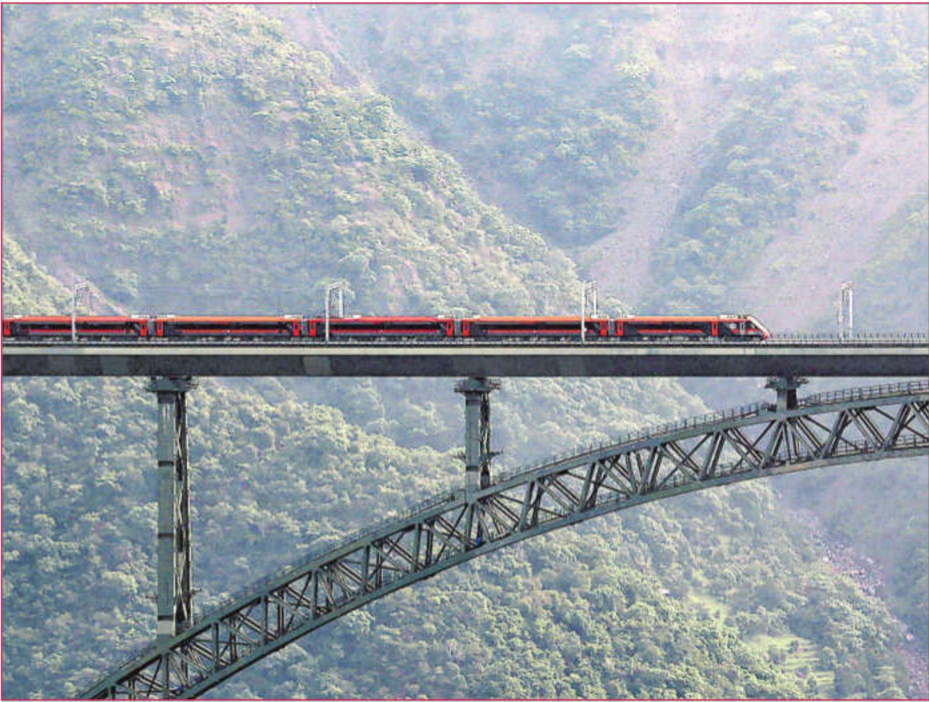
A Vande Bharat train runs on the railway track of the Chenab Bridge in Reasi on Sunday. The Vande Bharat Express successfully traversed the 359-metre-high Chenab Rail Bridge in Jammu and Kashmir, showcasing India's engineering prowess amid the monsoon challenges.
