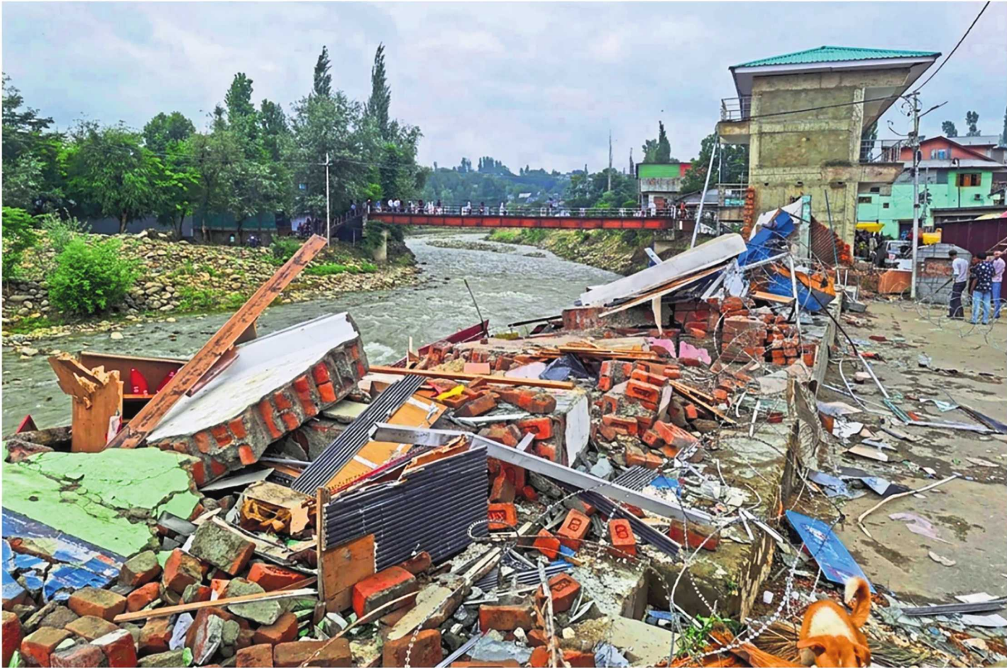
The debris of a shopping complex that was destroyed by cloudburst-triggered flash floods along the Sukhnag stream in Beerwah, Budgam district, on 21 July.
