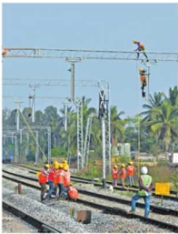
The four railway projects will expand the existing network by about 410km. MINT
