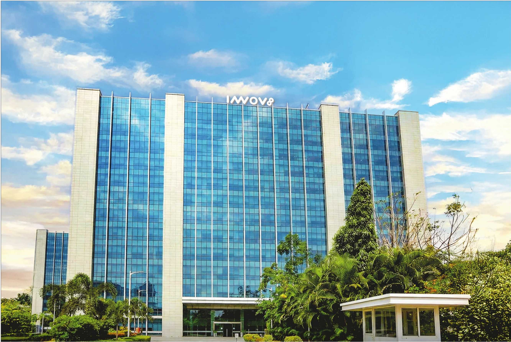
PRESTIGE TECH PLATINA, KADUBEESANAHALLI, OUTER RING ROAD, BENGALURU, KARNATAKA | GRADE-A TECH PARK | 100 M FROM THE METRO STATION
